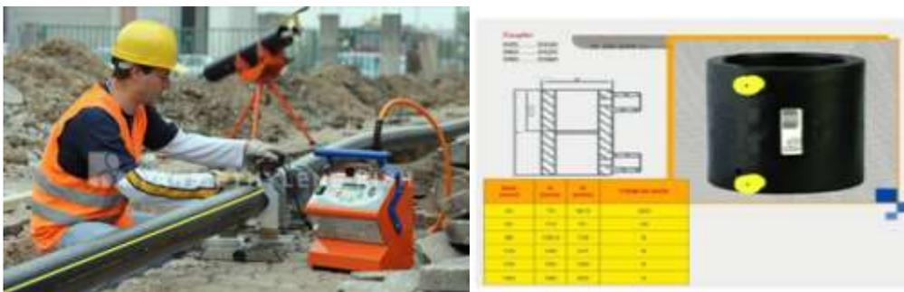
Figure 1. Electrofusion coupler and weld production equipment
