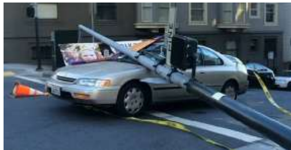
Figure 1. Lamp post collapse due to corrosion in San Francisco (2015)
