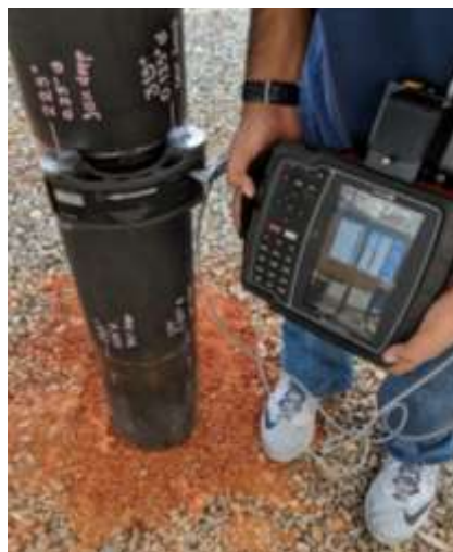
Figure 10. Lamp post inspection using Innerspec PowerBox H and MRUT MS Scanner (experimental trials)
